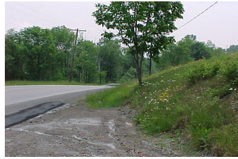
Before slope flattening
