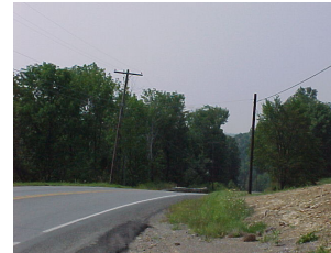
After slope flattening
