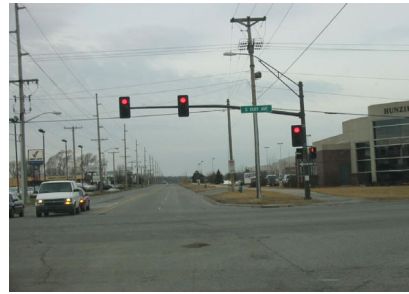
Treatments used in Springfield included installing a protected phase (left) and overhead signals (right).
